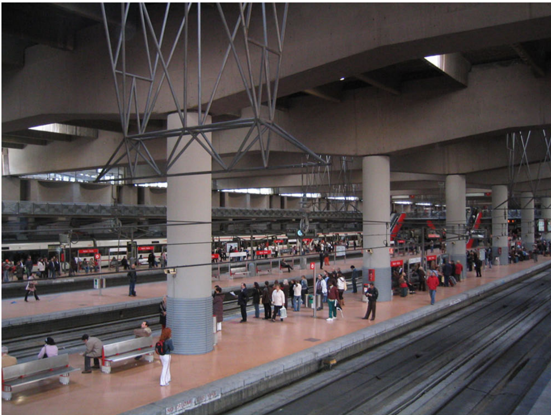
Atocha train station (Madrid, Spain).
