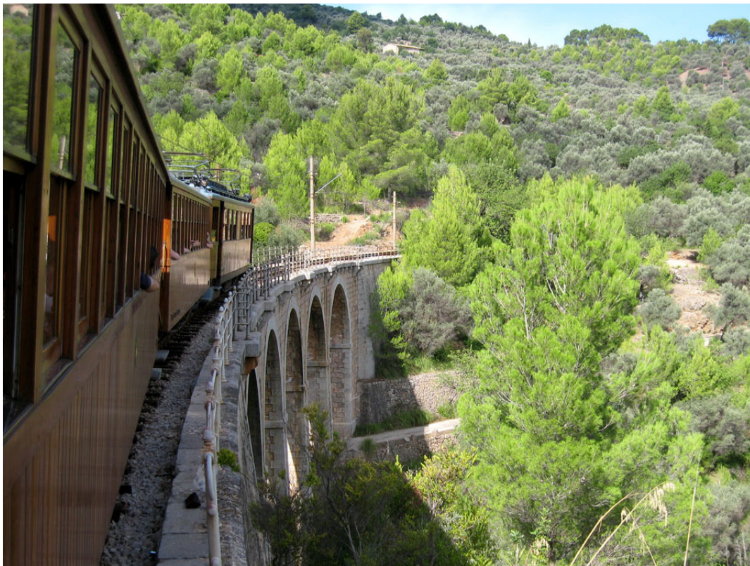
Cinc Ponts viaduct Mallorca, Spain
