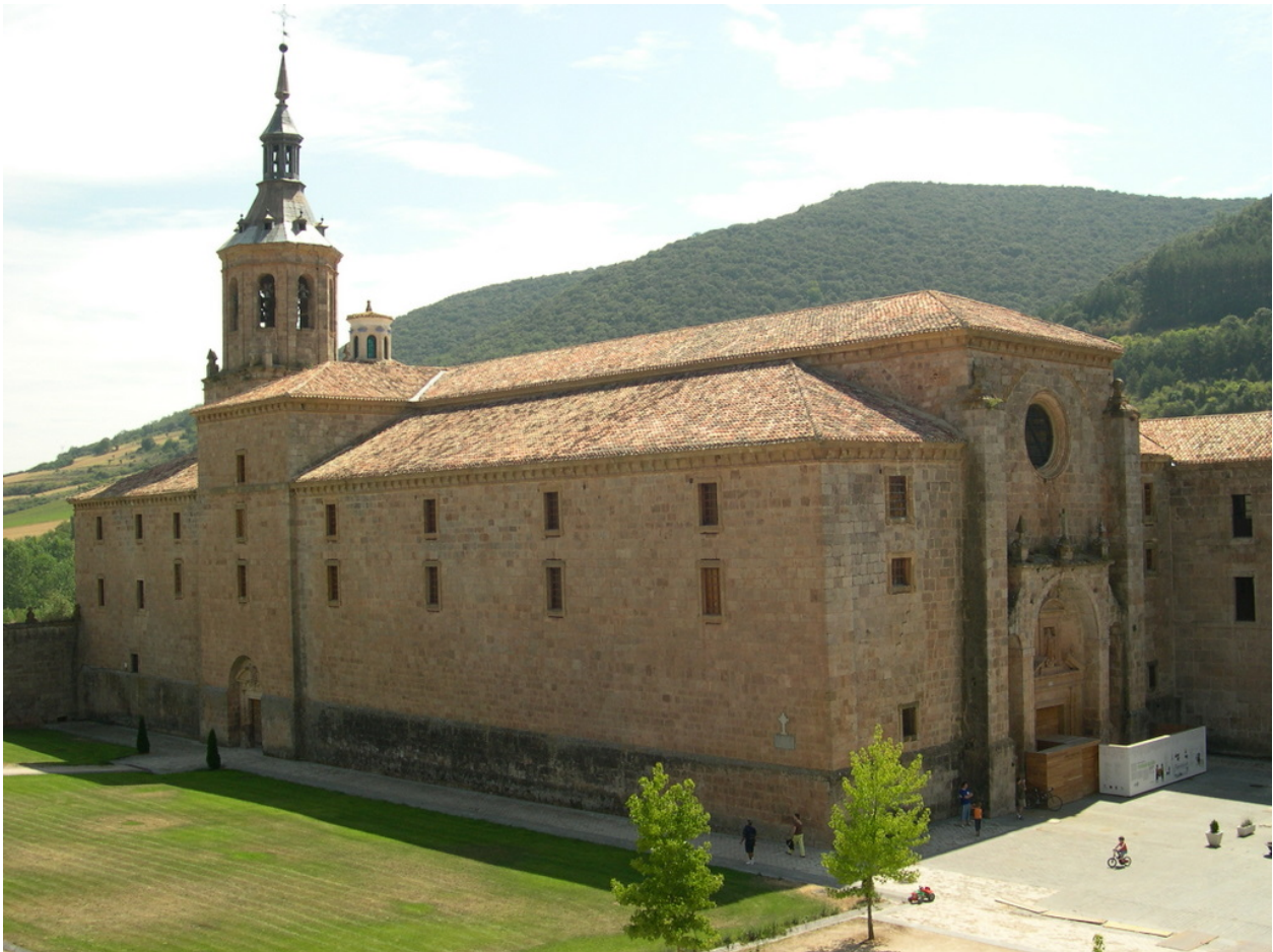
View of the Monastery of Yuso
